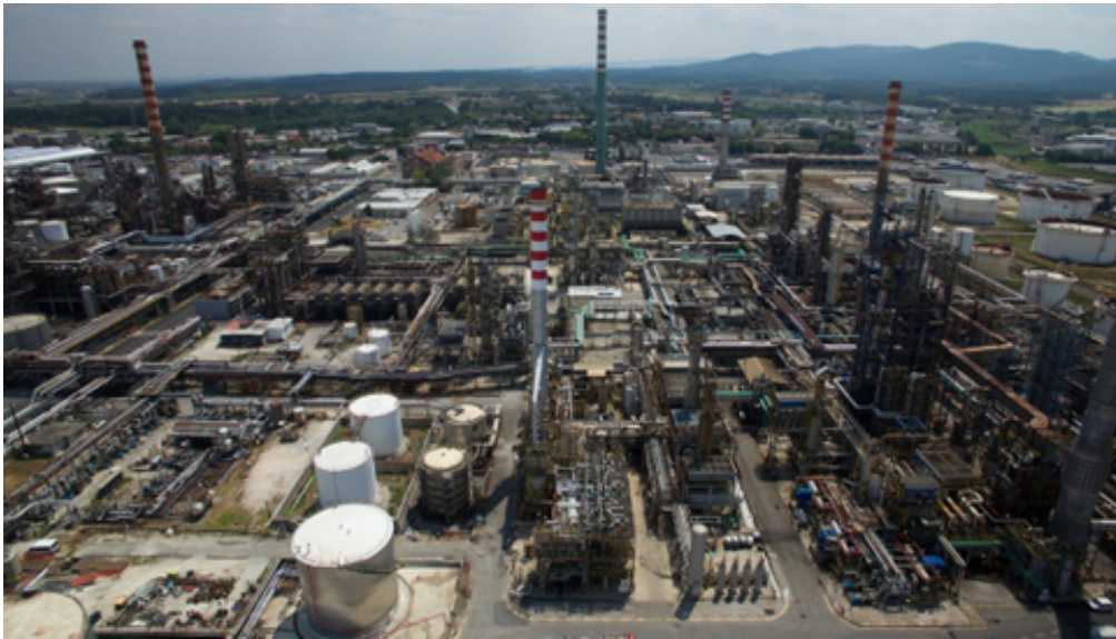
Fig. 1 - ENI refinery in Livorno. Source: ENI.
